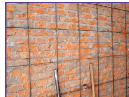
挂钢筋网外抹高强砂浆加固砌体墙
